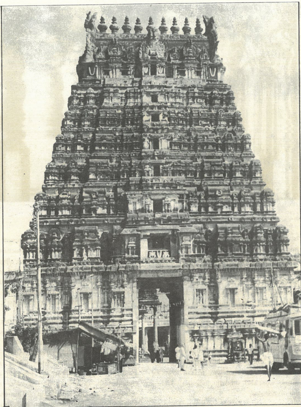
Gopura of Varada-rāja temple at Kāñchipuram
