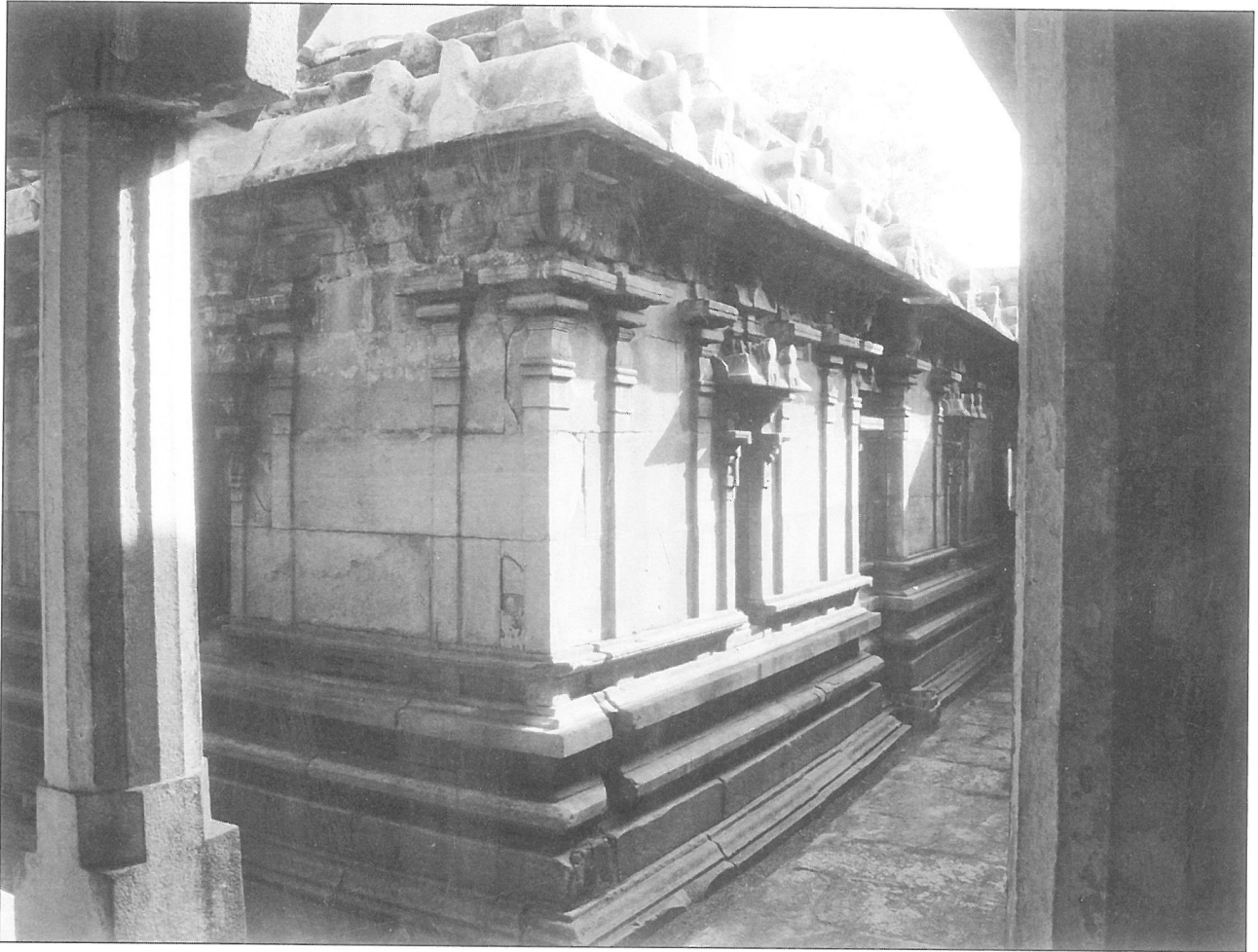
Outer walls of garbha-grha, view from north-west
