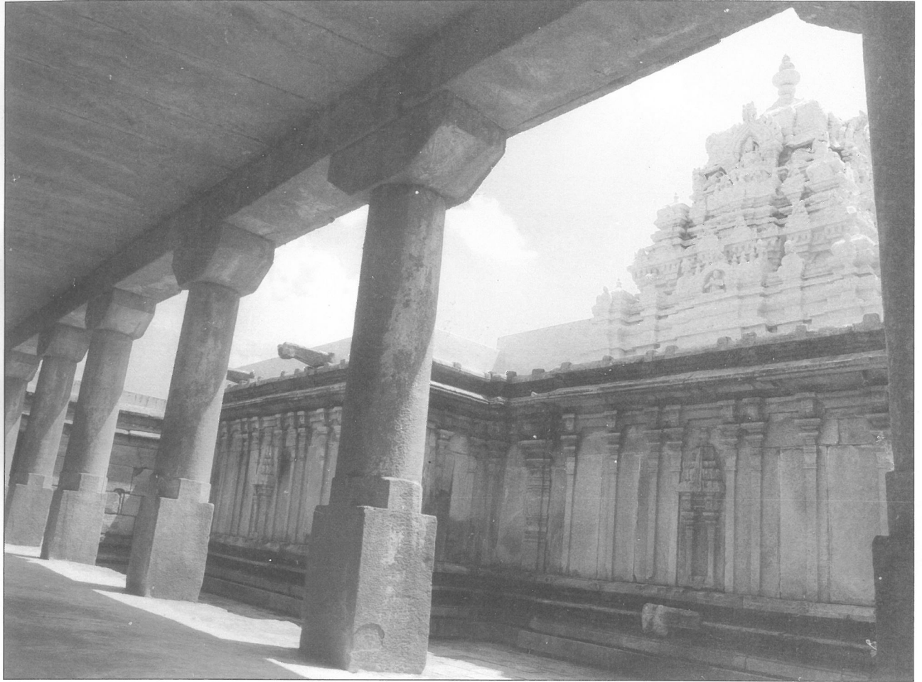
Vimāna-gopura, view from north-west
