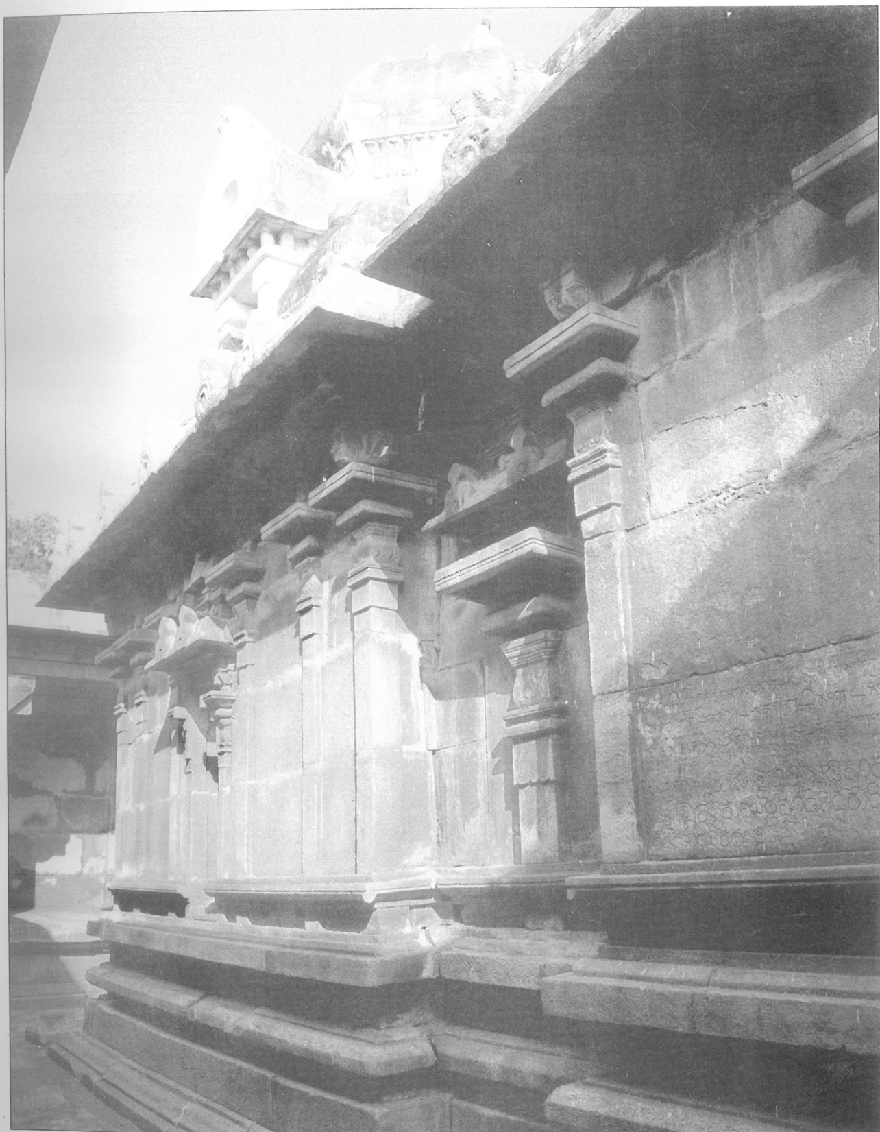
Vimānagopura and outer walls of garbha-grha; view from south-east
