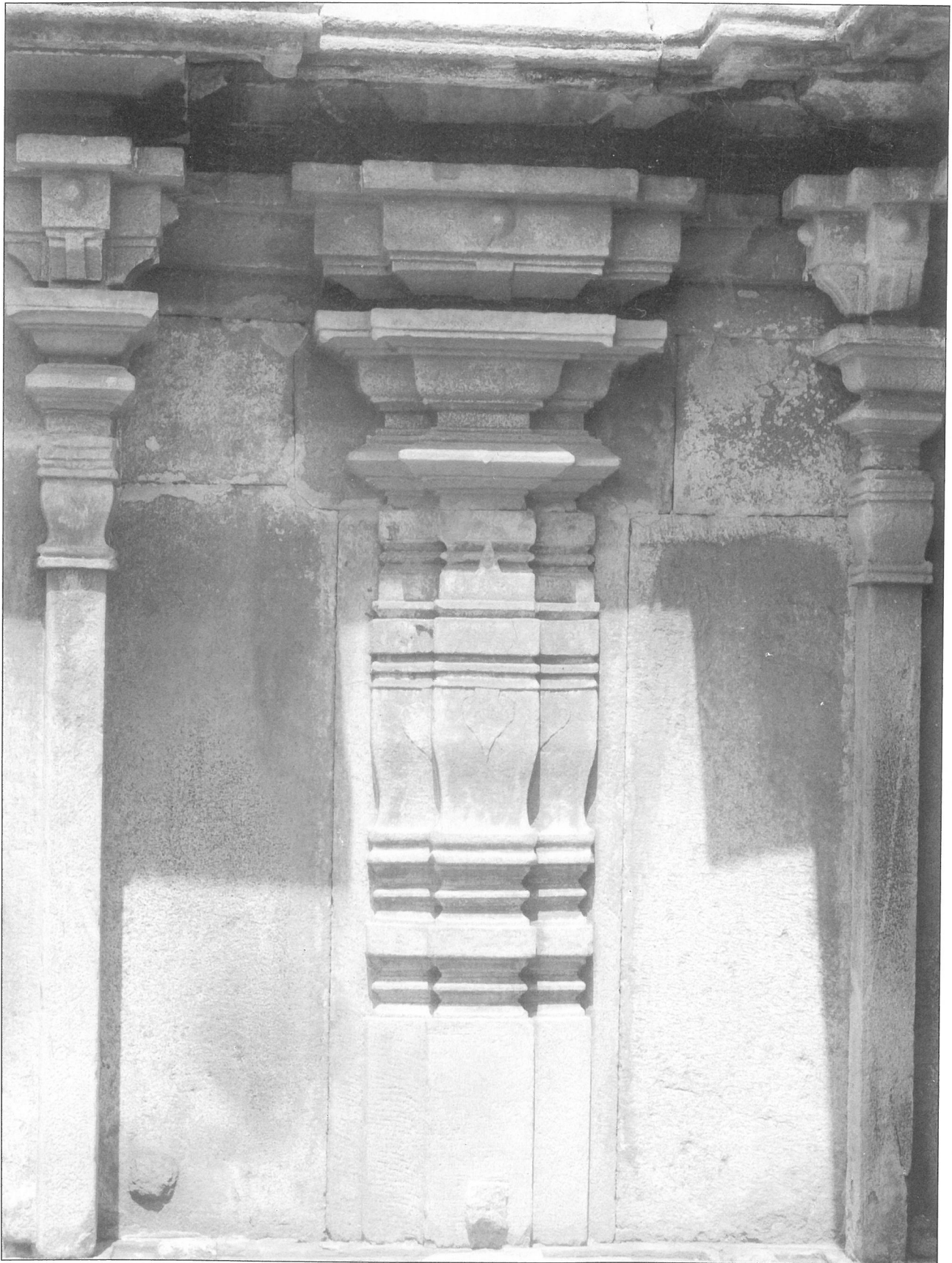
Details of Koshtha of niches on outer walls of the sanctum (garbha gṛha)
