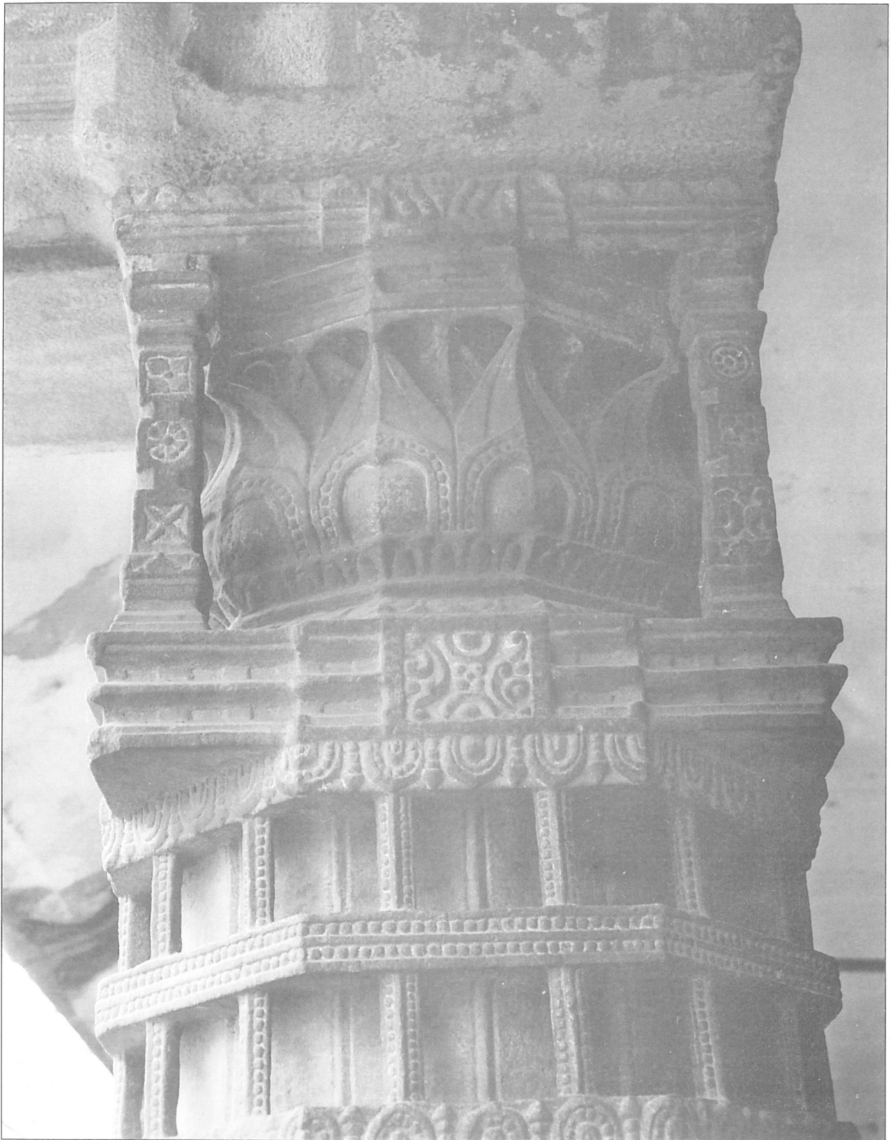
Close-up of another pillar
