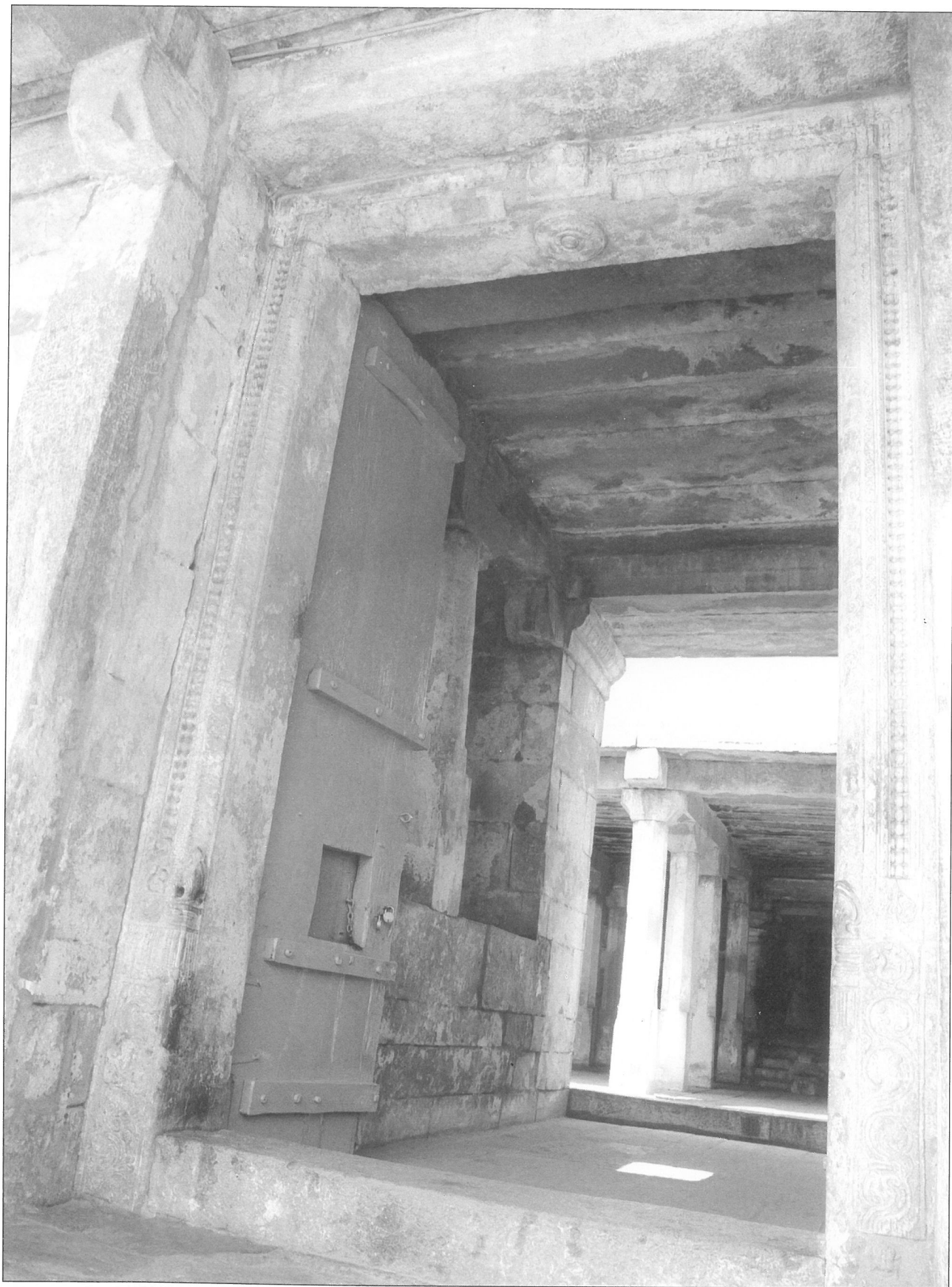
The main entrance (Mahādvāra)
