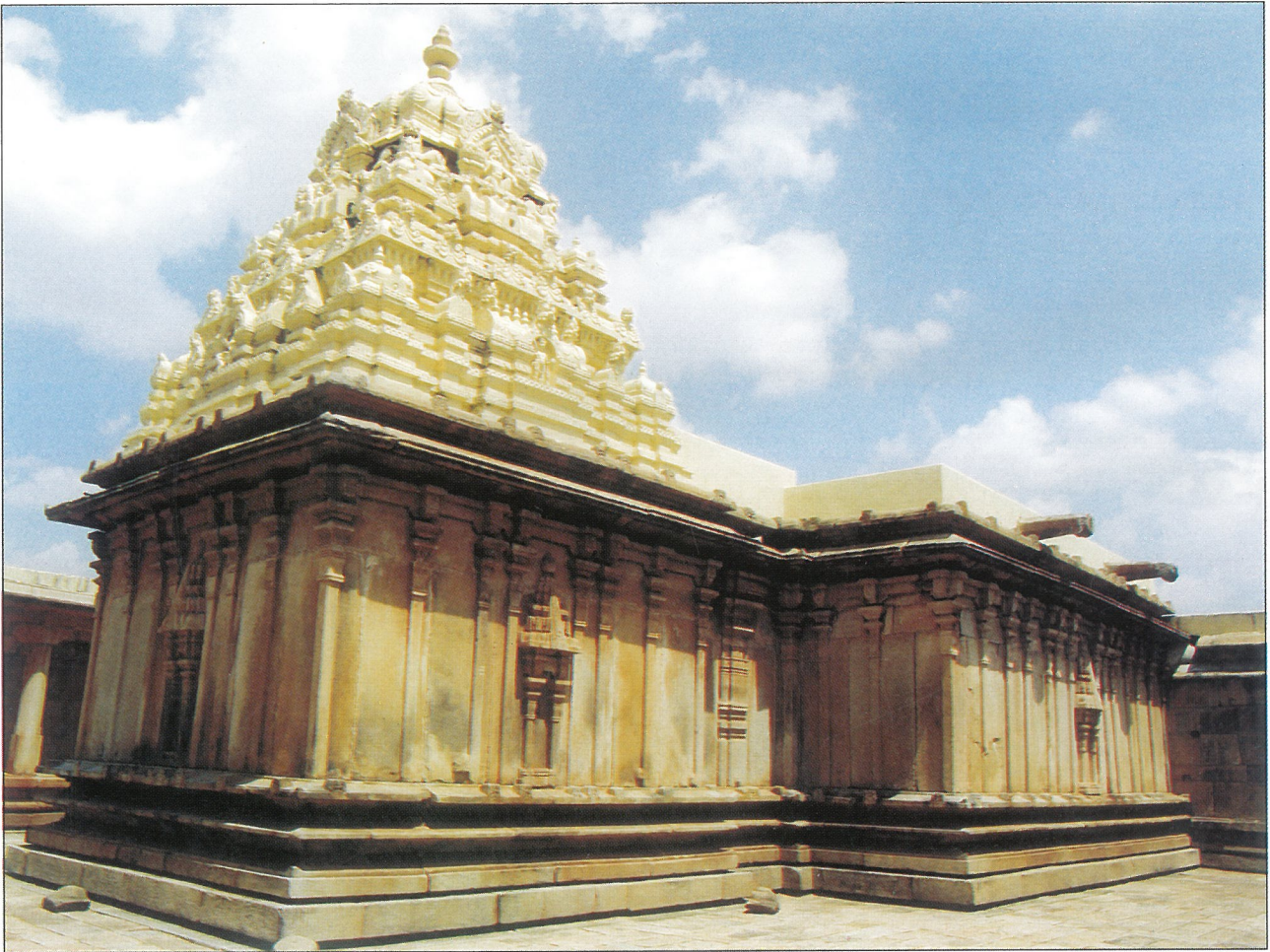
Vimāna-gopura, view from south-west
